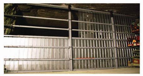
Reinforced frame system to resist deformation caused by close proximity blasting.
