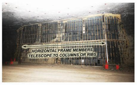
Horizontal supports telescope rib to rib and/or between columns to allow large structures to be constructed with relatively lightweight components fitting various entry sizes.
